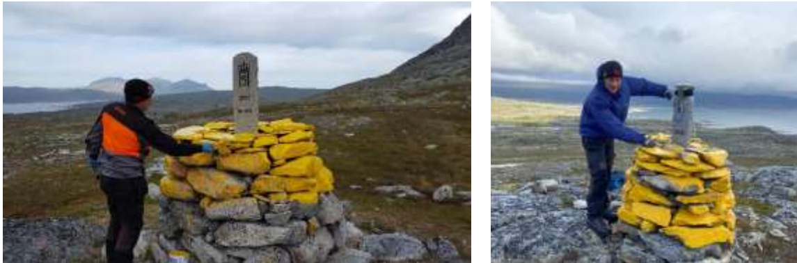
Figure 11: To the left a new heart stone is put into place and the yellow painting is refreshed. To the right Tor Erik Bakke is measuring the state boundary between Sweden and Norway with GNSS. (The Norwegian Mapping Authority 2022).
