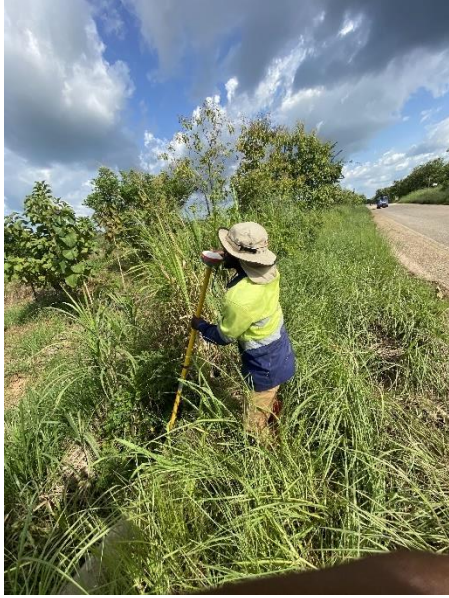
Fig. Identifying the pipeline route by RTK survey
