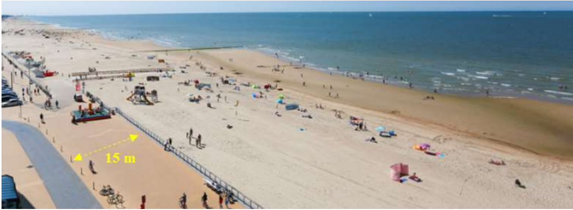
Figure 1. Mariakerke Beach and its typical seawall at mid-tide.
