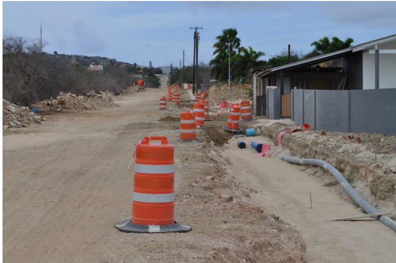
Fig. 8. Use case B3: Registration of utility lines (under above ground) and sewerage
