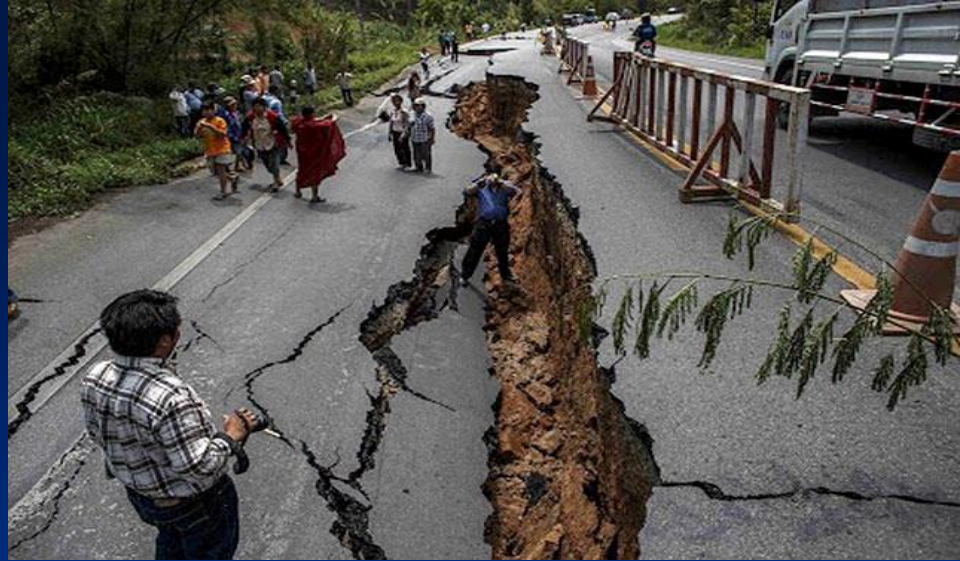
(2) Cracks in City Road
