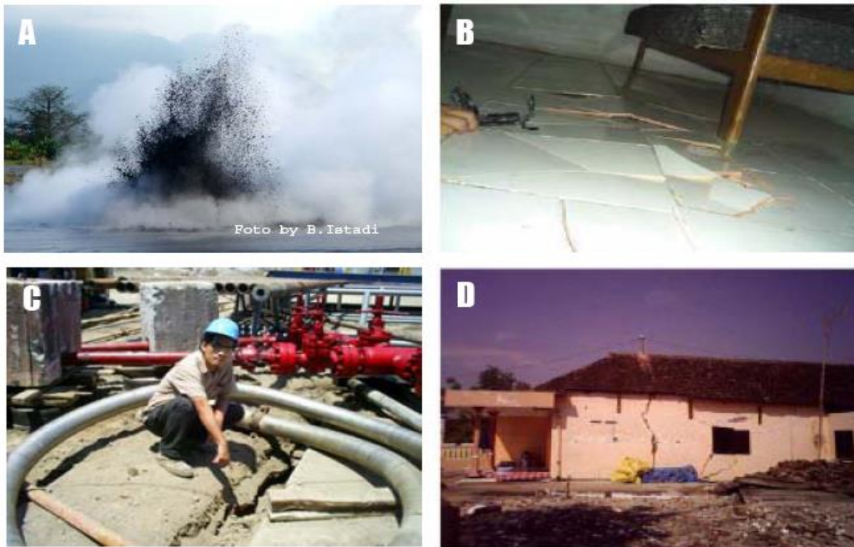
Figure 4 (A) LUSI mud volcano eruption, (B) crack on the floor, (C) crack on the ground around relied well-1, (D) crack on the house in Sengon Village
