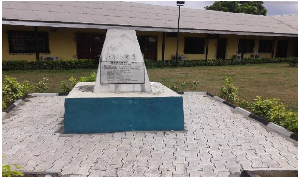
Fig 1.0: Specimen of a Typical Monuments as Survey Control Point RVOSG X1 (Source: Rivers State Office of the Surveyor General)
