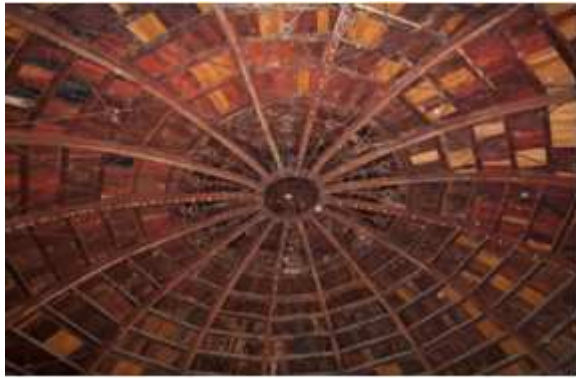
Figure 2 - Interior view of the dome
