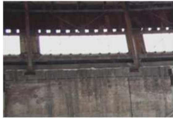
Figure 3 - Connection between ribbings and curb
