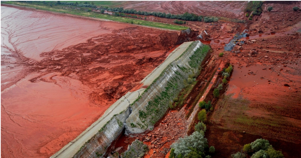
Figure 2.: The damaged dam of the reservoir
