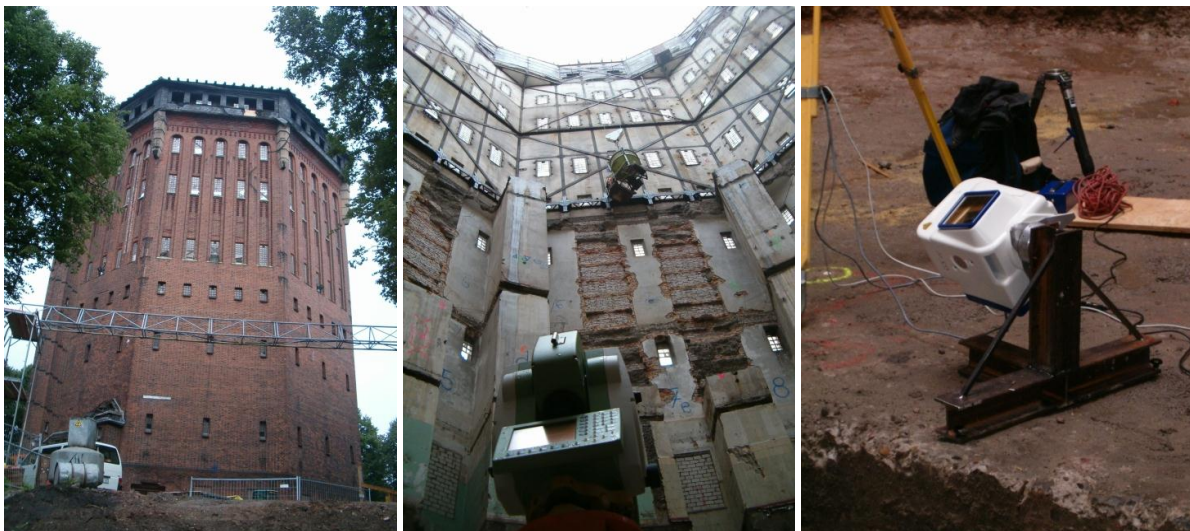
Figure 2: Former water tower at Sternschanzen Park in Hamburg: view at the external facade (left), interior view (centre), scanner GS100 on the special socket on the ground level of the tower (right)
