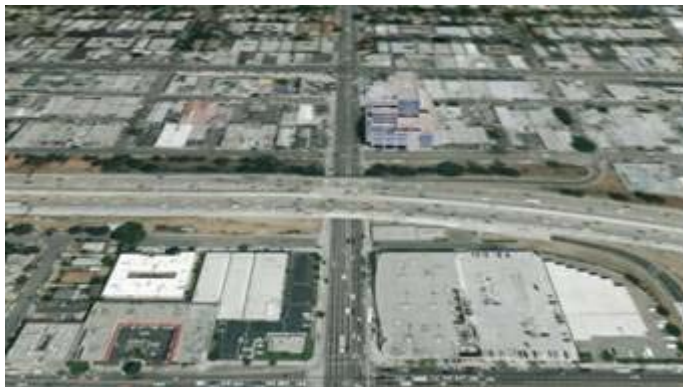
Figure 6: Bridge view (© Google Earth)
