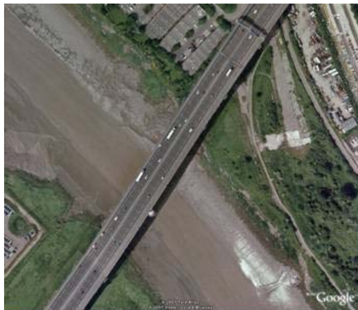
Figure 2. A Google Earth image of the viaduct.
