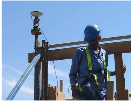
Figure 1: GPS and circular prism collocated
