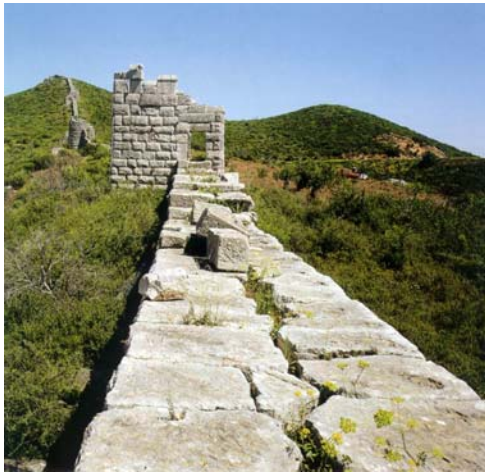
Fig. 2: View of the Walls in the West side
