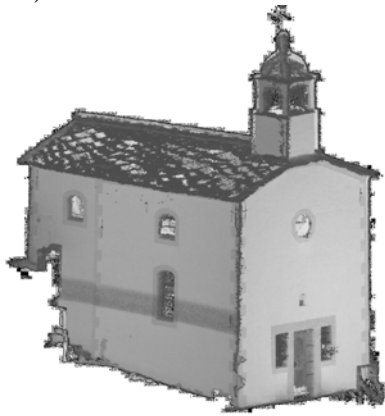
Figure 12a: Registered point cloud
