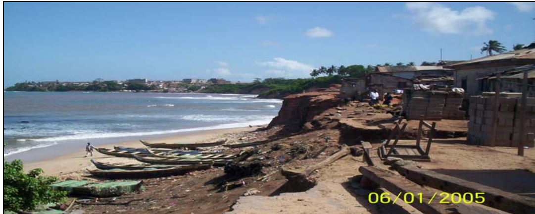
Plate 1: Serious Erosion Downdrift of Takoradi Port
