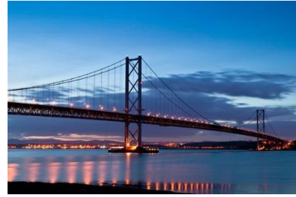
Figure 2 the Forth Road Bridge (Scotland, UK).
