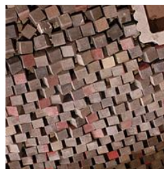
Fig. 5 Concrete blocks of the armour layer.
