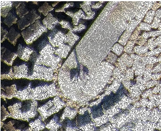
Fig. 22 Ortho and point cloud (top view) of the head of the breakwater.
