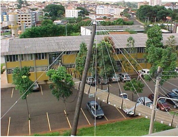
Figure 4. Cable-stayed wooden footbridge at the Sao Carlos Engineering School, USP
