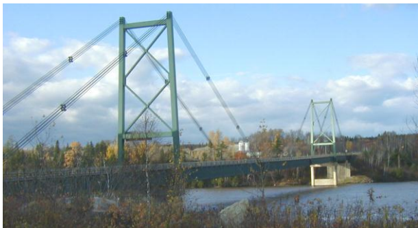
Figure 5. Hawkshaw Cable-Stayed Bridge, New Brunswick, Canada
