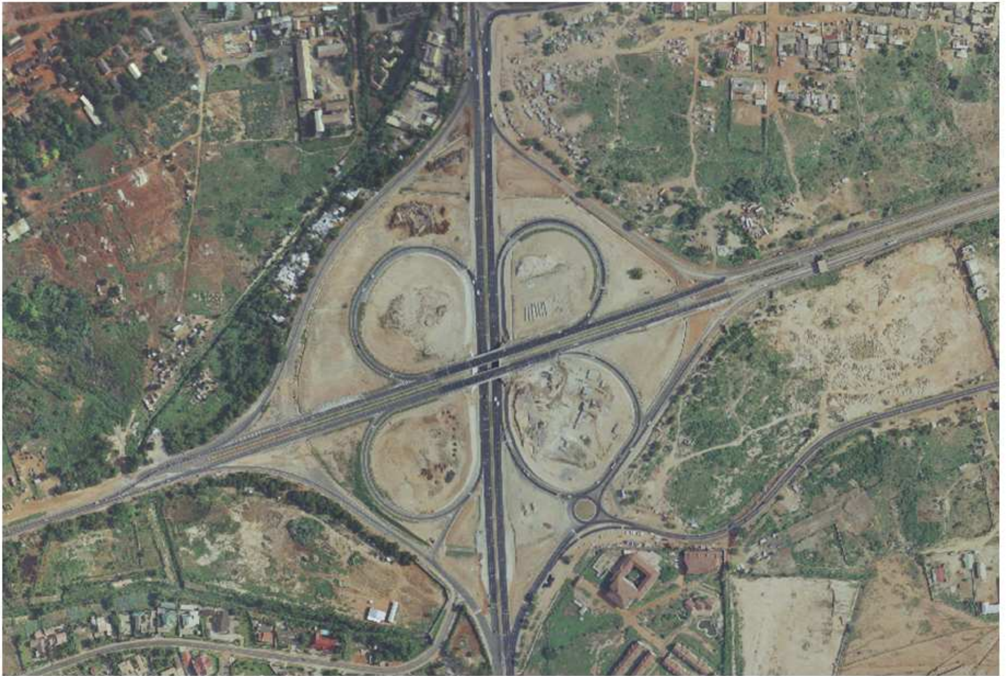
TETTEH QUARSHIE INTERCHANGE
