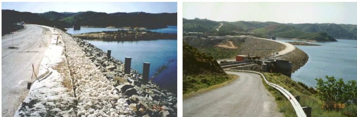
Figure 9 –Beliche Dam. Execution of the rehabilitation works
