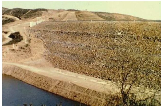
Figure 4 – Beliche Dam. Berm constructed on the upstream face
