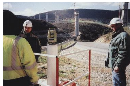
Construction of the Viaduc de Millau in 2003 with a laser theodolite.
