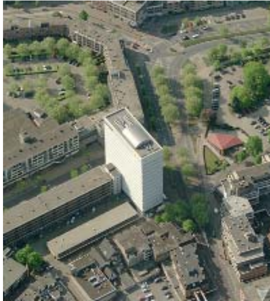
Figure 2 , Oblique view from the North on main building of Kadaster in Apeldoorn.
