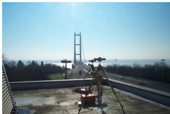
Figure 5: The two reference stations on top of the Humber Bridge board building with the bridge in the background
